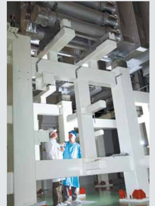
Framework for the pre-amp modules on CEA's Megajoule laser, used to recreate the conditions involved in nuclear fusion. Sagem is a partner in this program.
